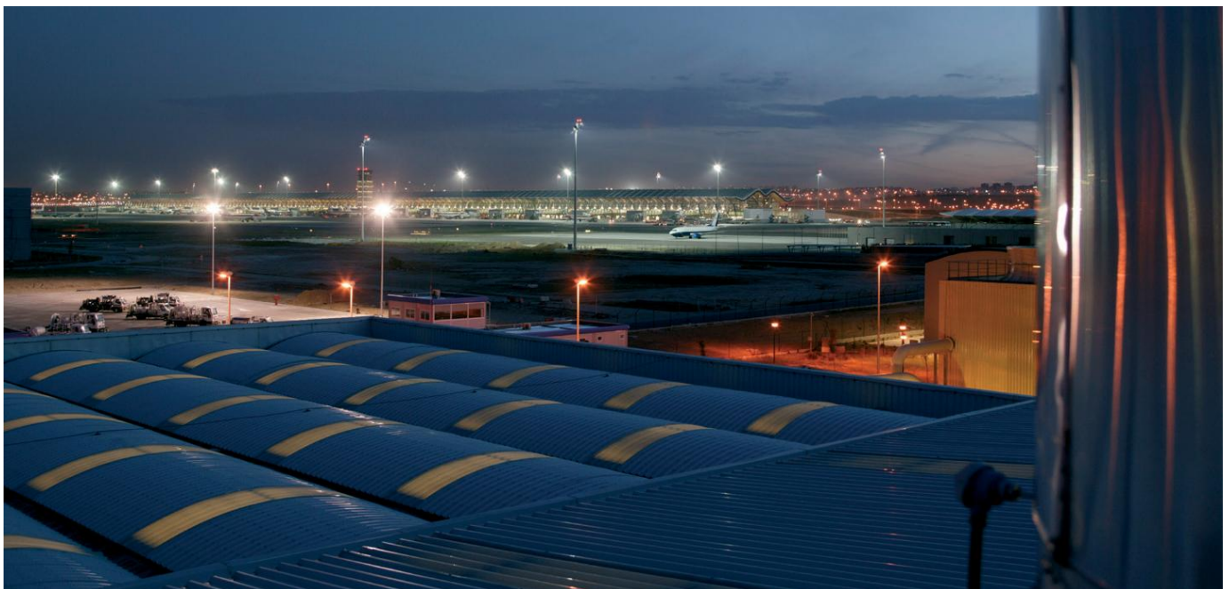
Fig. 17. Trigeneration plant at Adolfo Suárez Madrid-Barajas Airport. The plant is based on reciprocating engines fueled mainly with natural gas and has been ensuring the reliable supply of electricity, heat and cooling for the largest airport of Spain since 2005.
