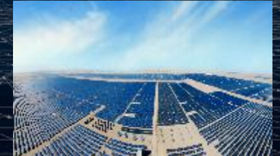
100% green power co-construction
