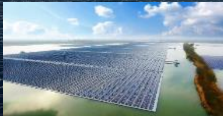
Floating solar plant 60MW @Huaibei, Anhui
