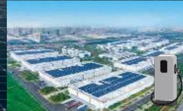
Solar access in campus @Dongguan, 17.5MW, PV + charging
