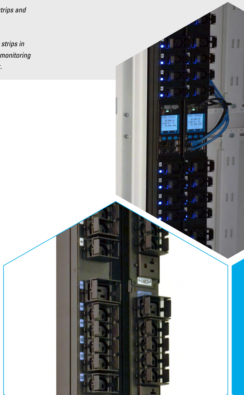
Figure 1: PDUs and Power Strips are used to distribute power into ICT racks and cabinets.
