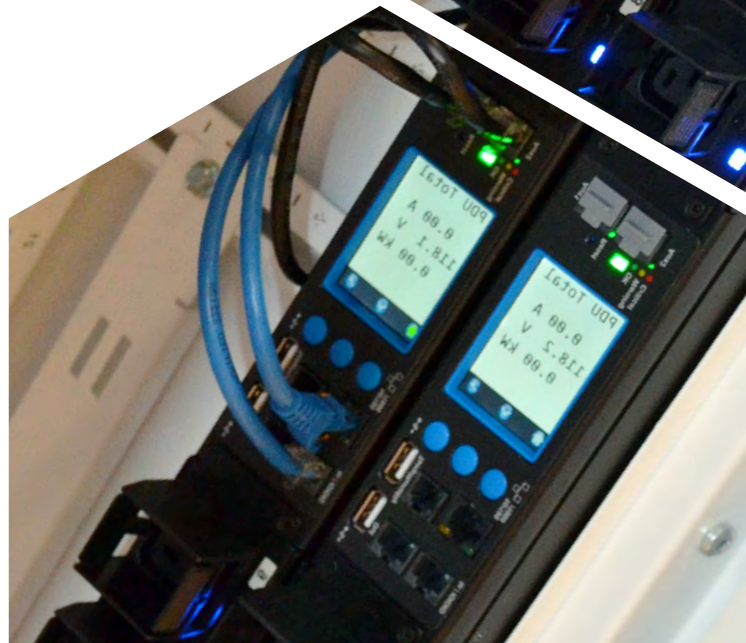
Figure 3: Vertical PDUs and power strips are typically used in cabinets and racks that are 6' (2 m) high, 23.6" (600 mm) wide, and 42U or larger. Horizontal PDUs and power strips are used in wall-mount racks and cabinets.
