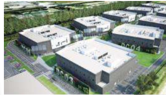
DATA CENTER MILAN
